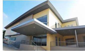
IPC Sucat Data Center
