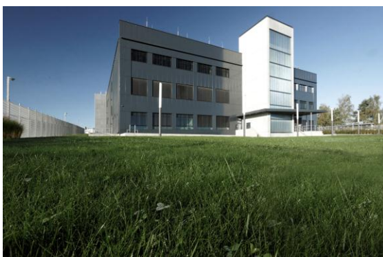
Datacenter in Zurich
