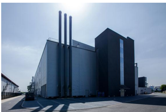
Datacenter Campus in Frankfurt
