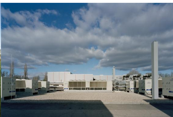
Datacenter in Berlin
