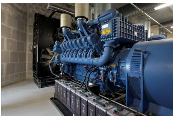
Generator facility of Datacenter in Frankfurt
