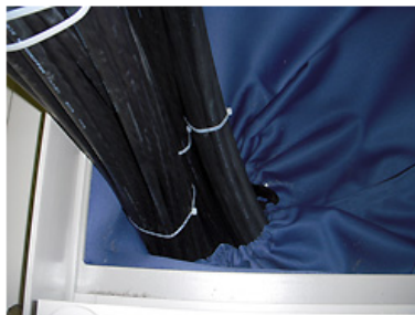
Trapping cool air under the double floor using a drawstring seal
