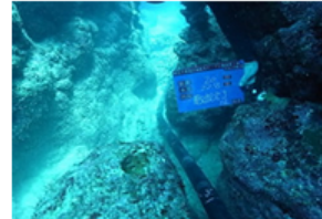
Cables are laid in natural ocean floor trenches
