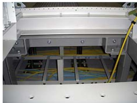
Wiring layout with dual-walled structure (underfloor)
