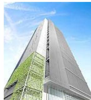
earthquake as strong as the Great East Japan Earthquake or the Great Hanshin Awaji Earthquake. The data center is also equipped with high-efficiency power generating equipment and an advanced air-flow management system capable of reducing energy use by up to 35%. As a result, the PUE (Power Usage Effectiveness) is under 1.45, giving the data center one of Japan's highest levels of environmental performance.
