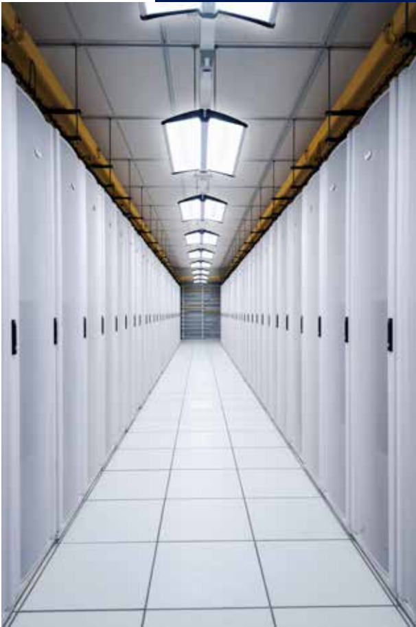
54U Rack and Smart Lighting
