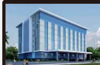
India Mumbai 5 Data Center
