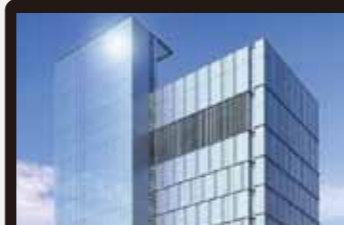
Japan Osaka 5 Data Center
