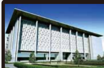
Thailand Bangkok 2 Data Center
