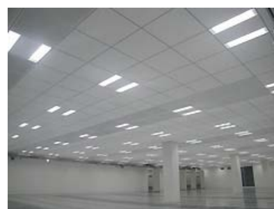
LED lights at a data center
