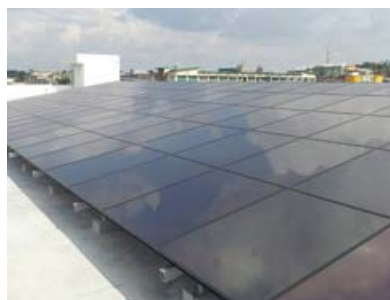
Solar panels installed on the rooftop of the Data Center building in Malaysia
