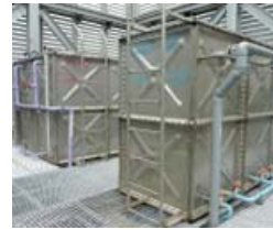
Surrounding water tanks with shade mesh protects them from direct sunlight.
