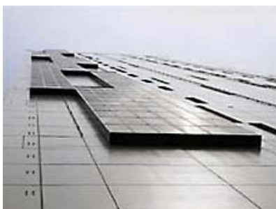
Solar panels installed at Tokyo No. 5 Data Center
