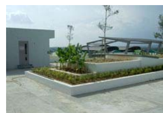
Rooftop gardening of the Malaysia data center
