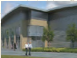
United Kingdom Slough 2 Data Center
