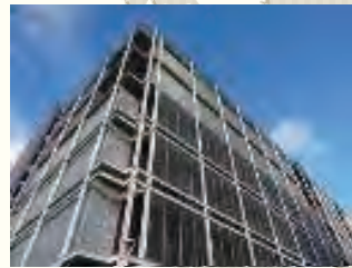
Japan Tokyo No. 6 Data Center
