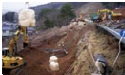
Cable restoration work
