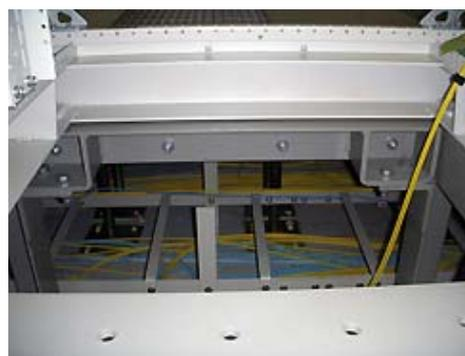
Wiring layout with dual-walled structure (underfloor)
