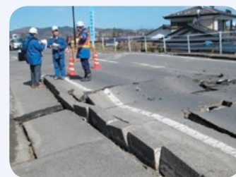
Digging up a severed cable
