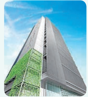
The Tokyo No. 5 Data Center
