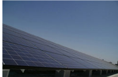
■ Solar panels installed at a data center in Tokyo
