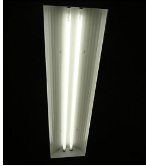
■ Fluorescent light bulb with reflector
