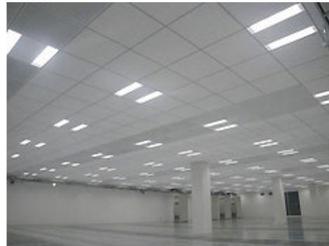
■ LED lights at the data centers
