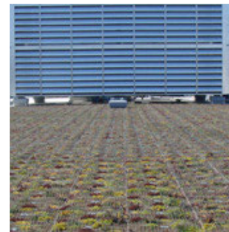
■Rooftop garden installed on a data center building in Tokyo
