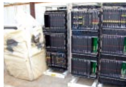
■ Dismantling and recycling equipment at premises of intermediate treatment contractor
