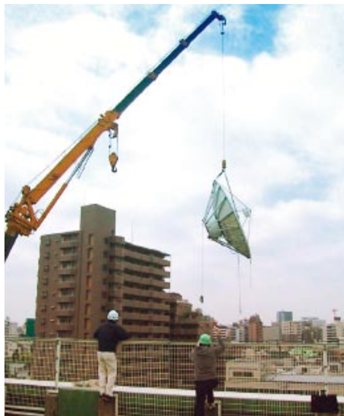
■ Removing satellite communications equipment
