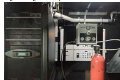
Fuel cell-based UPS
