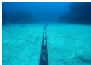
We lay cables on the sand, away from coral reefs
