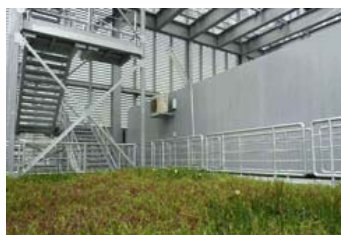
Rooftop gardening of the Singapore data center
