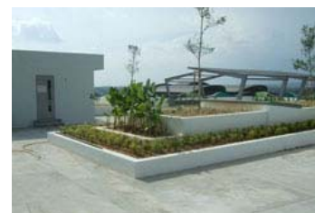
Rooftop gardening of the Malaysia data center
