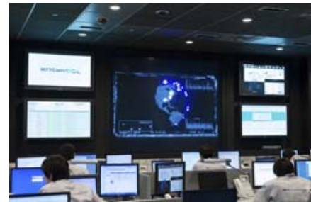
Security Operation Center
