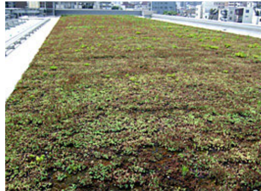
■ Rooftop Garden on Telecommunications Building
