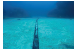
[ Cables laid on sand to avoid coral reefs ]
